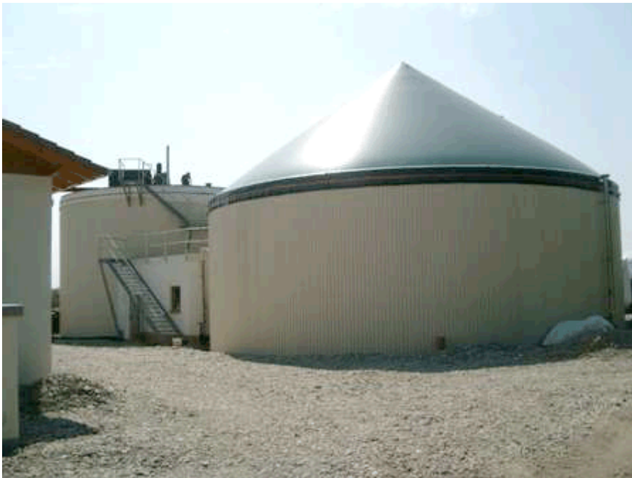
digestion of energy crops
